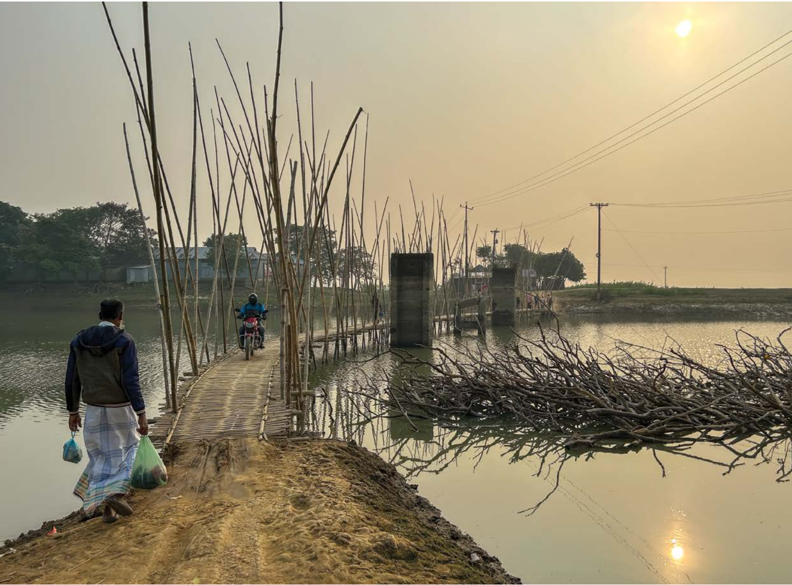
Infrastructure is fragile and needs investment.
