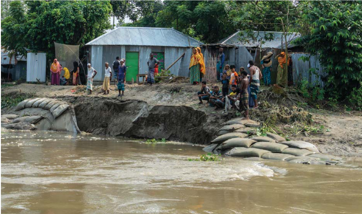
People gather to witness the flood defences being washed away.
