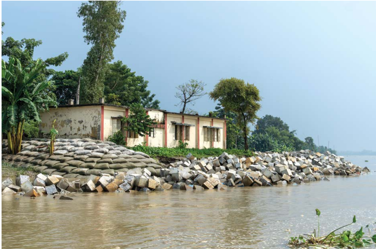
Geo-bags and blocks are placed in a bid to save a school just metres from the collapsing riverbank.
