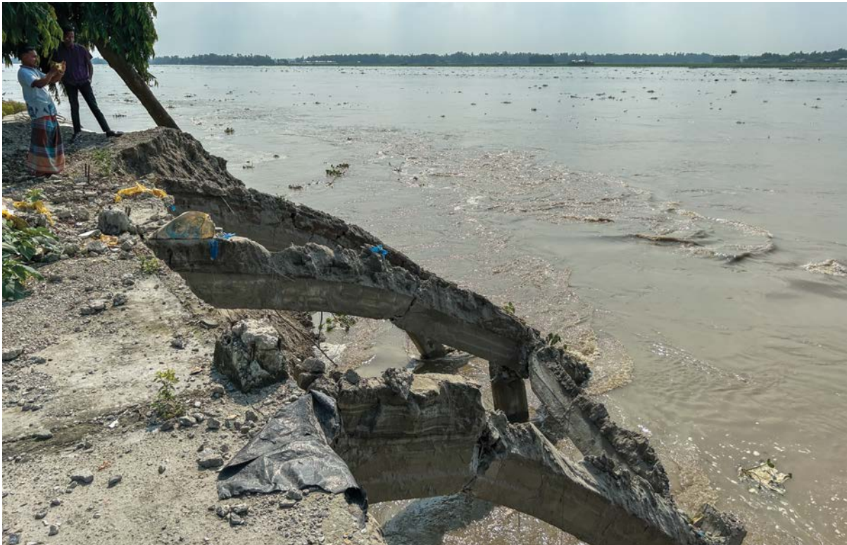
Community institutions, including clinics, markets, offices, madrasas, flood shelters, and mosques, have already fallen into the river, such as this primary school.
