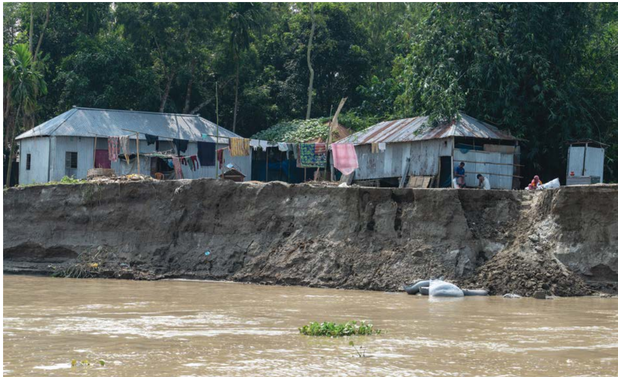
Rapid erosion tears away Kurigram’s fragile char land, where entire settlements vanish as the river shifts without warning.
