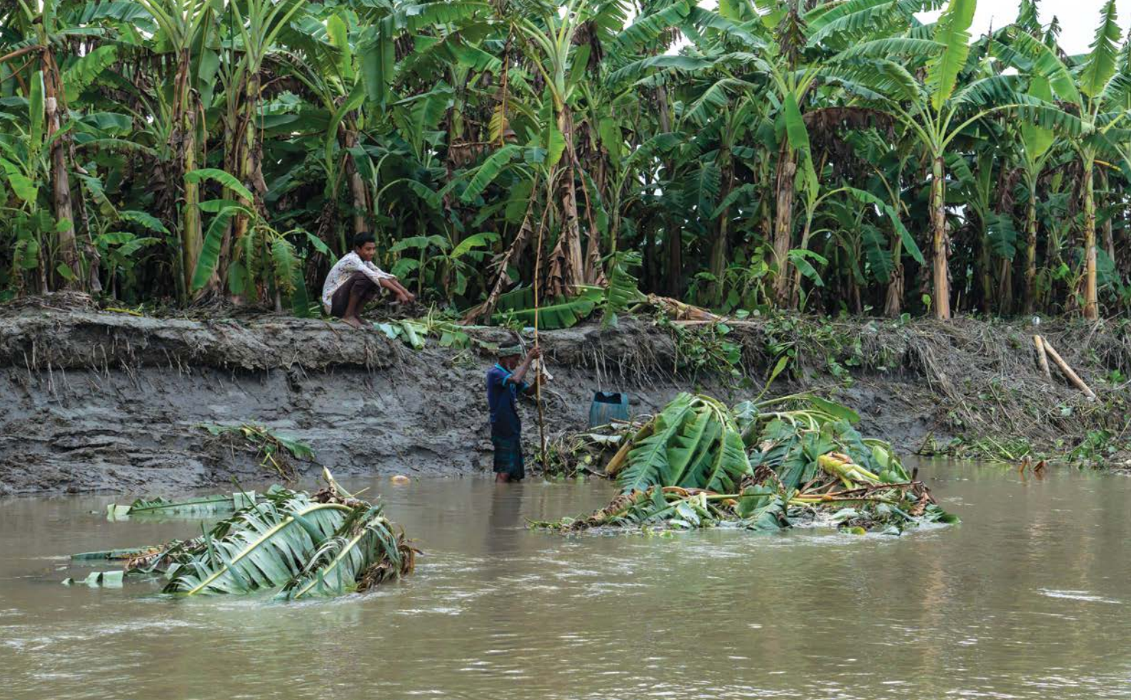
Villagers reinforce the bank with sandbags and bamboo in an effort to slow the erosion.
