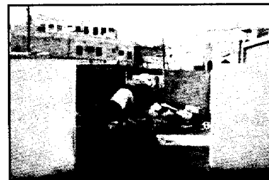
A masonry enclosure for a waste collection point
