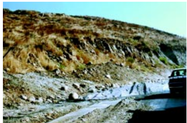
Figure 3: Typical denuded slope alongside an urban road that is in constant danger of eolic as well as hydrologic erosion. (Road that leads to airport from bus terminal.)
